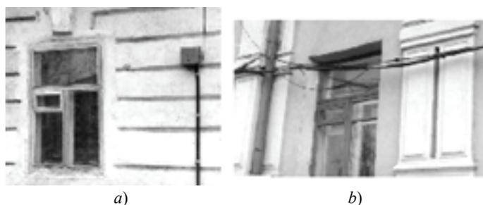
**Pic. 3 Telephone switchbox (*a*) and laying of cable lines along the facade of a building (*b*)**
